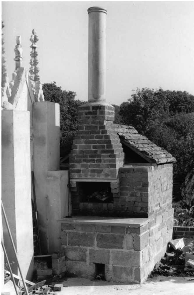
A photograph of the author's oven at Allaleigh shortly after its completion in 1988. No external render has yet been applied, and the roof is exiguous. I now have a lean-to canopy springing off the gothic screen on the left-hand side to protect both the oven and the work space. (Photograph, Clare Paroley)
