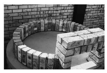
Lay a course of soldier bricks (bricks built up on end) to form the base of the dome. Use the 1,4 m circle as a guide to mark the position of the outside surface of this course of bricks. Allow the mortar to set and gain strength for at least 24 hours before any further work is done.
