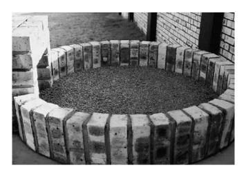
Spread out a 20 – 25 mm layer of 5 to 7 mm stone over the oven floor to provide some insulation for the oven floor. The volume of blinding stone required is approximately 35 *l*. The top surface of this layer is carefully levelled to provide a flat surface for laying the clay paving bricks. The stone layer is tapered to be thinner near the door to limit restricting the door opening when laying the paving bricks. Those in the doorway should be laid in bedding mortar to keep them in position.
