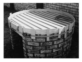
To make removal of the formwork easier, a thin layer of release agent should be applied to the inside of the side forms as well as the top surface of the base timber. Spray and Cook, Vaseline or cooking oil have been found to be satisfactory.
