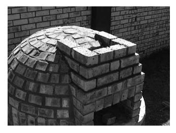
The chimney is constructed by building up above the oven door and over the top of the oven dome. Two low parallel 'walls' form the sides of the chimney. The side walls extend over the top of the dome.
