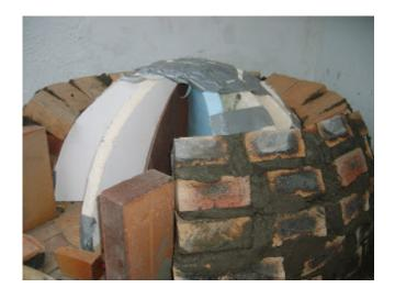
The mouth was difficult to do, in the end I put to fire bricks on end and then put two 4cm corner pieces of iron and fitted half bricks onto it.
