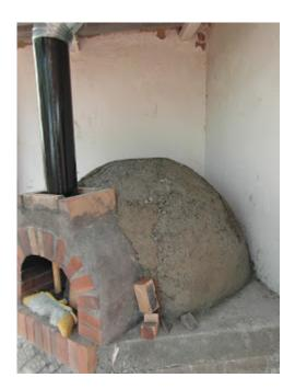
Then I covered the dome in Rockwell insulation, fixing it all with chicken wire, which I anchored with screws into the base. I covered this with concrete with a couple of trowels of lime mixed in to help it stick. I made quite a dryish mix and pushed it into the mesh. My husband said it wouldn't stick but it did. When it had dried I covered it in cement.
