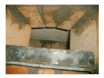
I fitted a piece of iron in the opening for the chimney pipe to sit on.
