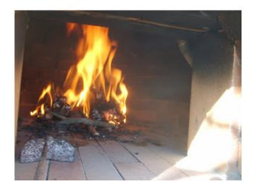
Before advancing any further I let the cement dry for a couple of weeks and then built fires in it for a couple of weeks until I brought the temperature up to 300c.
