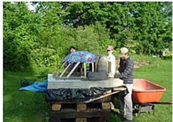
We first positioned the oven doors which we salvaged from an old woodstove. For the oven floor we laid out soapstone we got free from a local woodstove manufacturer's throw out pile -- we hit a good day. For the frame that will support the oven walls we ripped an 8 foot 2" x 4" into 1/8" thick strips. We added some branches for extra support and cloth on the top to keep sagging through the openings to a minimum. The frame will be burned out later.
