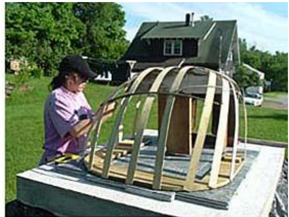
We built a frame over the foundation and poured concrete for the oven base. It's 5-1/2" thick.
