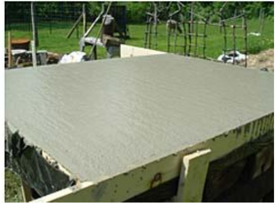
We built a frame over the foundation and poured concrete for the oven base. It's 5-1/2" thick.
