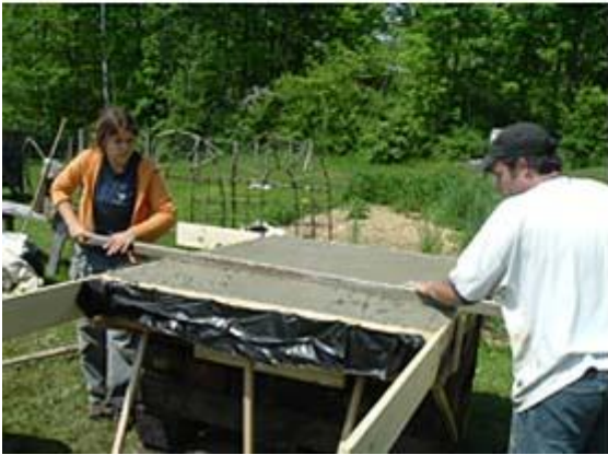
We built a frame over the foundation and poured concrete for the oven base. It's 5-1/2" thick.
