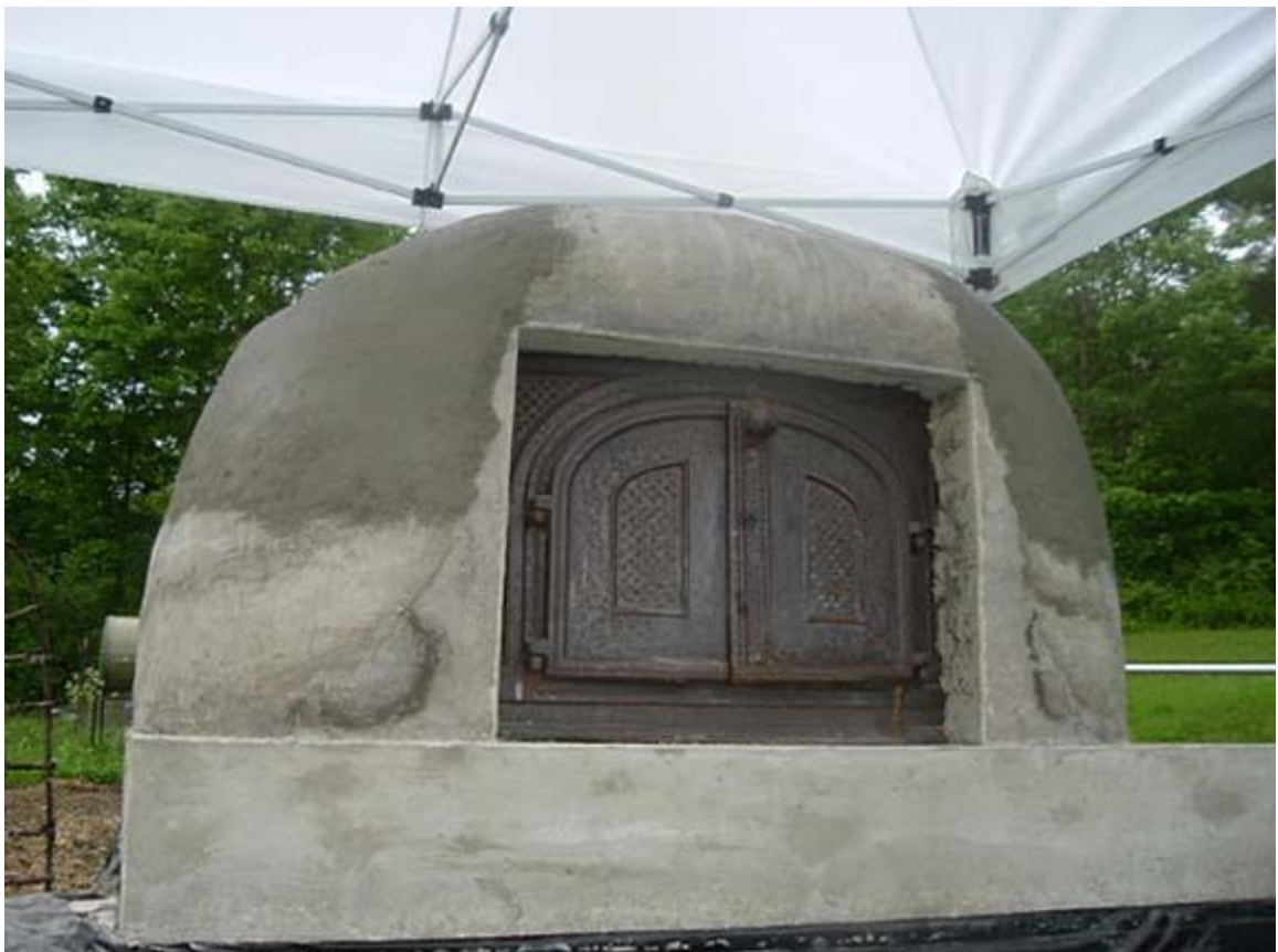
This is the finished oven before burning out the interior frame.
