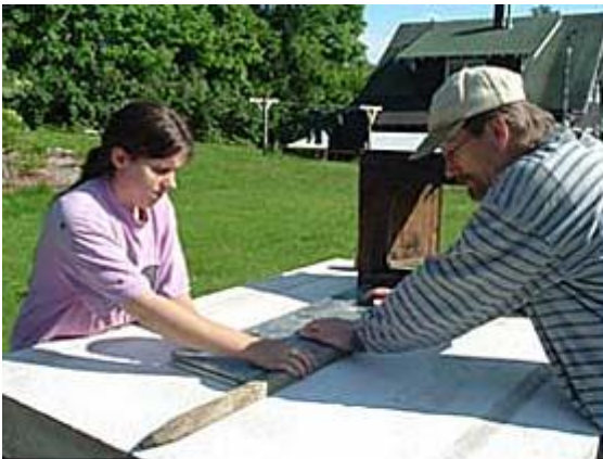
We built a frame over the foundation and poured concrete for the oven base. It's 5-1/2" thick.
