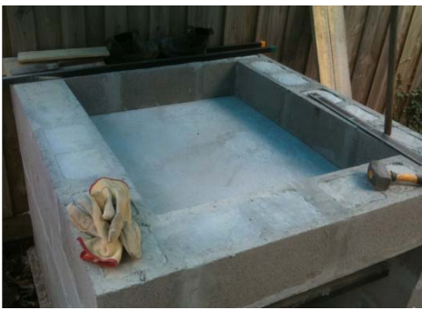
DAY 2 – The oven floor 16. Drop in 15mm cement sheet
