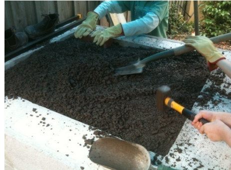
17. Fill with crushed rock and packed down hard.
