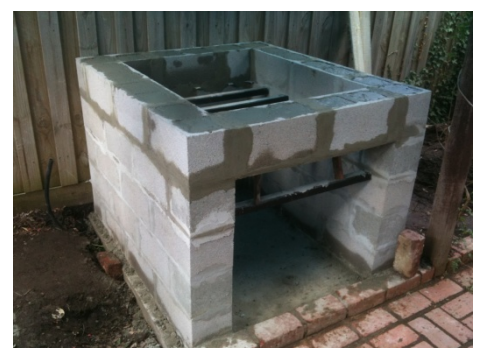
15. Ready for next stage. That's the end of day #1
