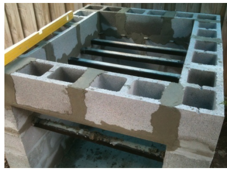
11. Could fill the besser bricks with concrete which prevents movement and reduces cracks in the mortar so I have been told. Also could put reinforcement bar inside the bricks. I didn't. Mine's still standing 😊
